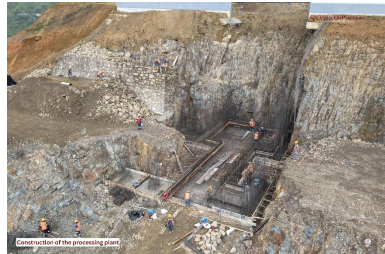
Construction of processing plant at El Domo. Source: Silvercorp
