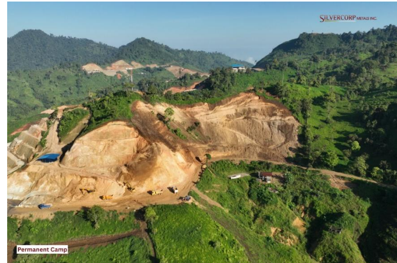
Construction of permanent camp at El Domo. Source: Silvercorp
