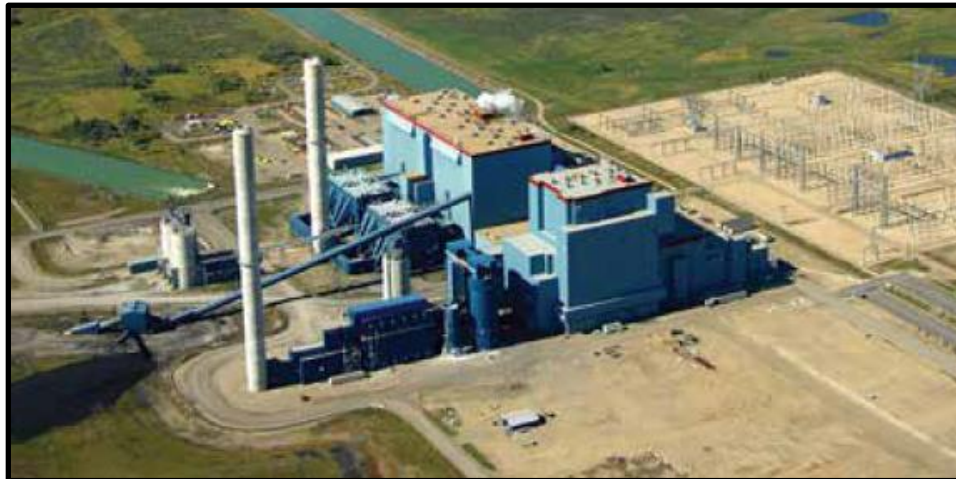
Genesee Power Plant
